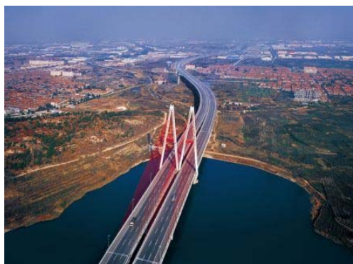
A bird view of Qingdao-Yinchuan expressway, Qingdao part
